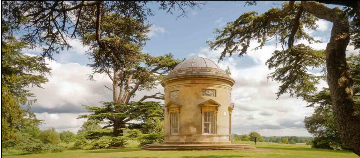
Capability Brown's Panorama Tower at Croome
